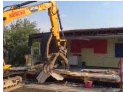
Holly Classroom... gone. Floor coming up.
